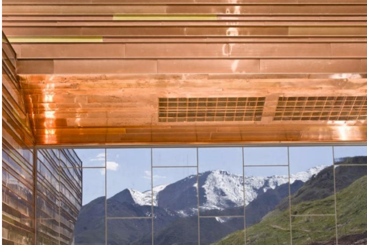
Figure 3.12: Interior glazing view of the Museum of Utah
