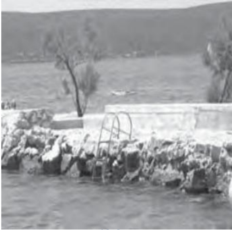
Figure 1.1 Artificial rocky bathing platform in Croatia, plus (inset) a typical ladder access facility
