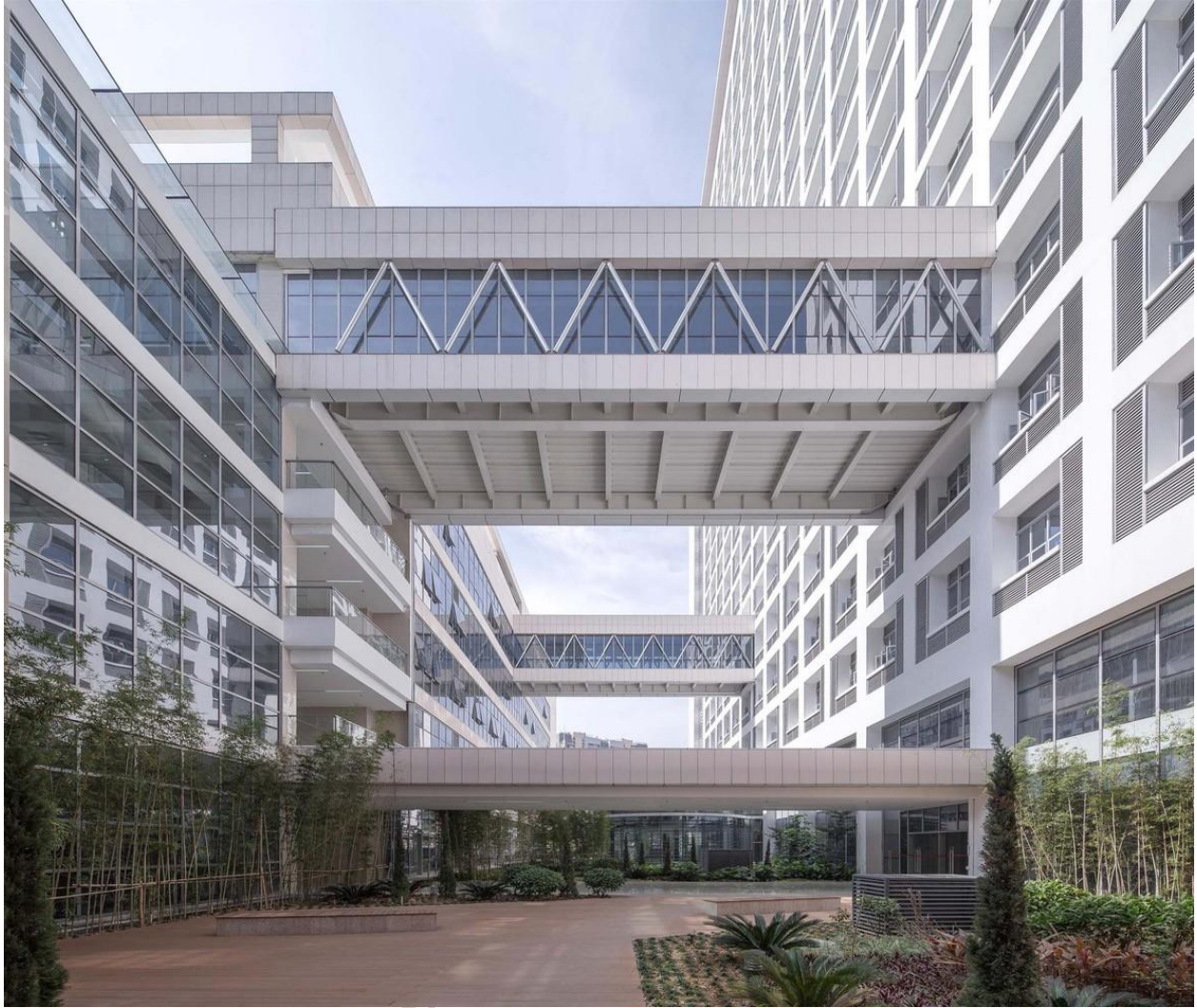
Figure 7 Shenzhen Bao'an Hospital elevation. Source: Archdaily.com
