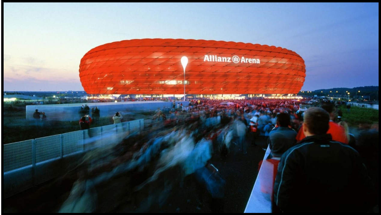
Fig 3.4: The Allianz Stadium, Munich.
