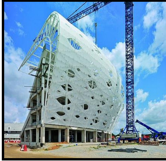
Plate 3. 2: View of the Stadium Showing the Crescent Steel Beams.
