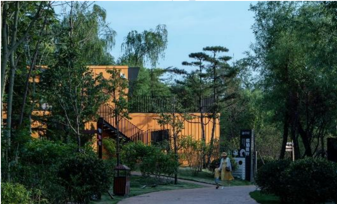
Figure 3.11: showing the stacking of shipping containers on each other Source: Researchers fieldwork
