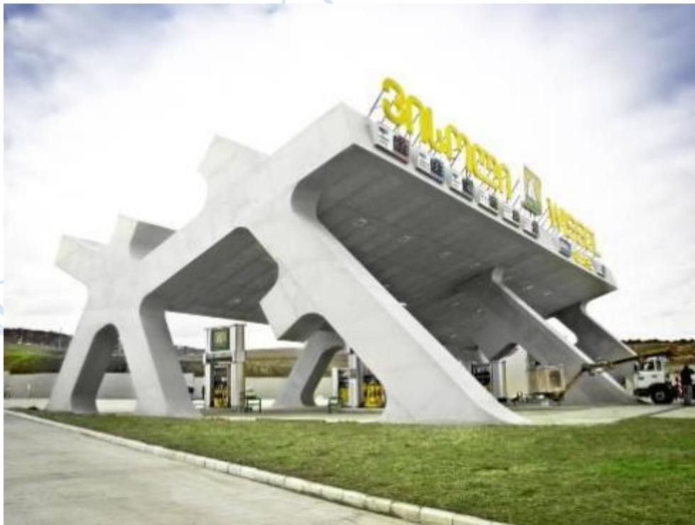
Figure 3.25: showing the filling station on site Source: Researchers fieldwork
