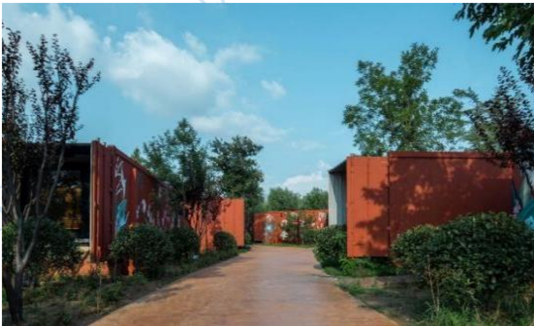
Figure 3.9: showing the arrangement of the shipping containers Source: Researchers fieldwork
