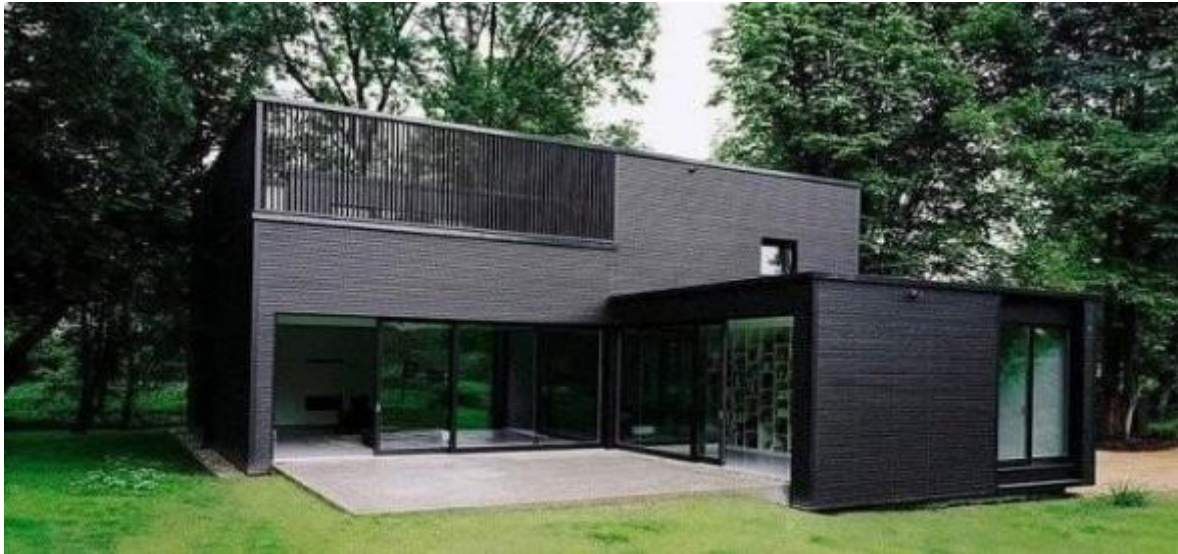
Figure 2.3: Highly modified shipping container home
