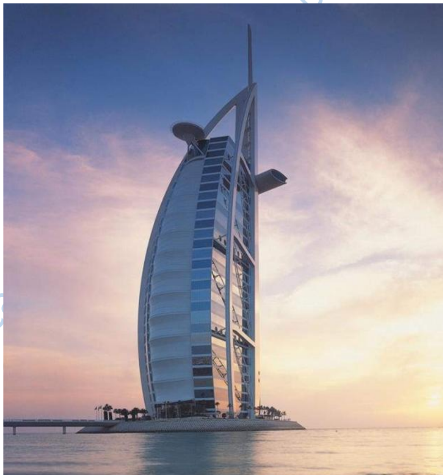
Plate 3.8: Exterior Facade of Burj Al Arab, Dubai (Source: www.canva.com )
