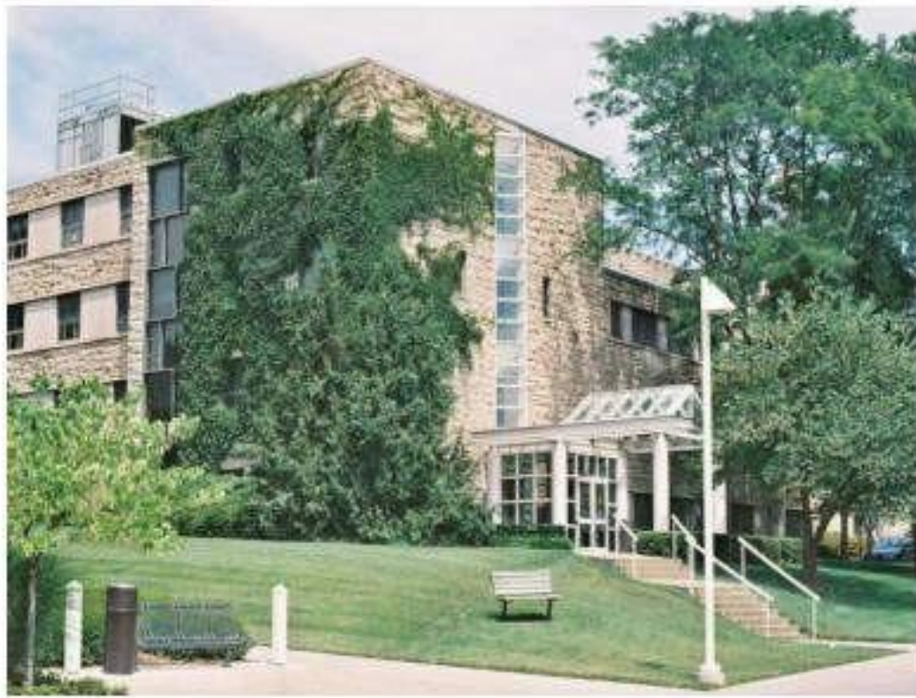
Plate 2.4: Good use of climbers and trees to reduce penetration of heat into the building, Rockhurst University, Kansas City, U.S.A. (Source: Ogunsoye, PrucnalOgunsoye, Adegbe, 2005).
