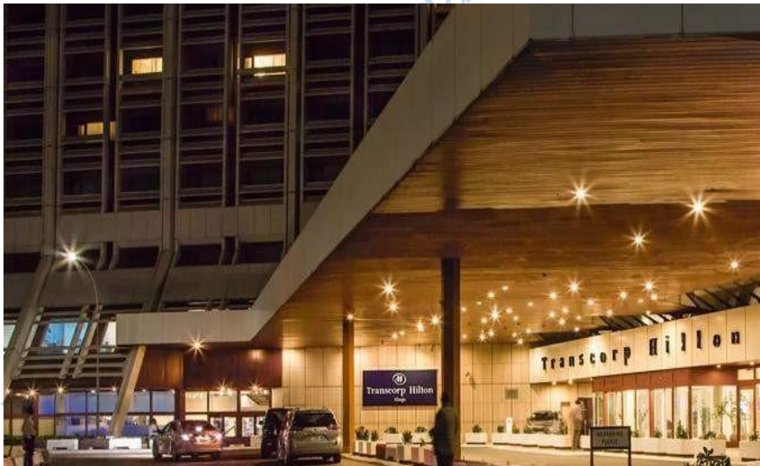
Plate 3.6: Grand Entrance at Transcorp Hilton Hotel Characterized by Canopy, Also Serve as Shading device (Source: Authots field work, 2024)
