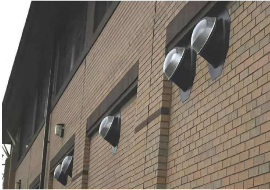
Plate 2.5: Sunlight tube captures day-lighting from the exterior walls of a building (Source: www.solatubes.com , 2014).
