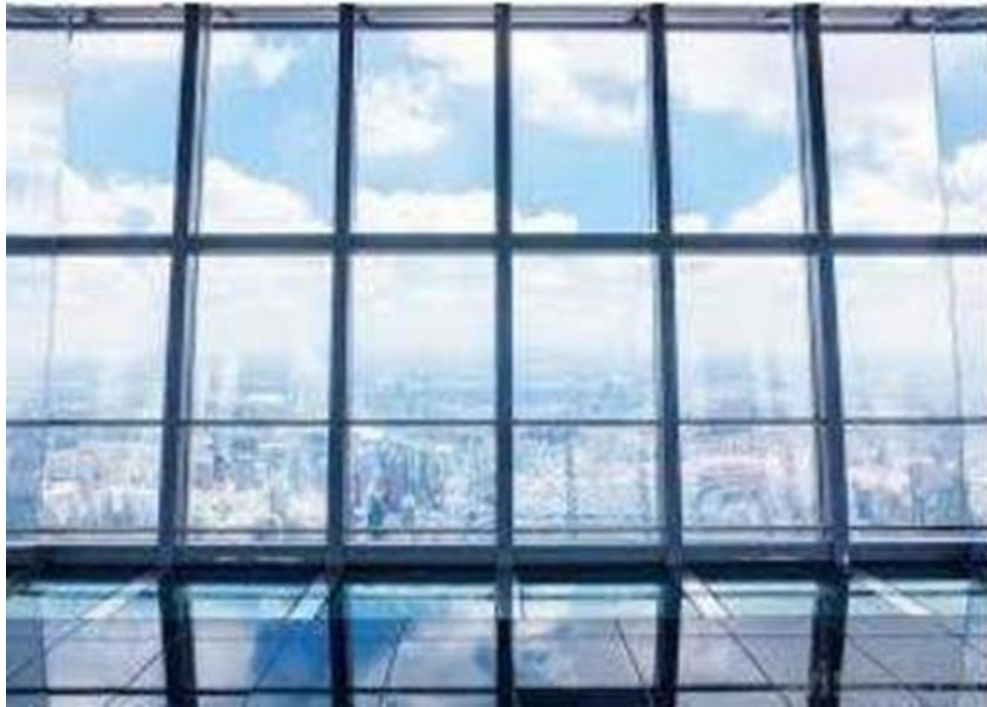
Plate 2.3: Use of solar reflective glass to enhance the cooling of the building interior (Source: www.smarthousingmanual.com , 2002).
