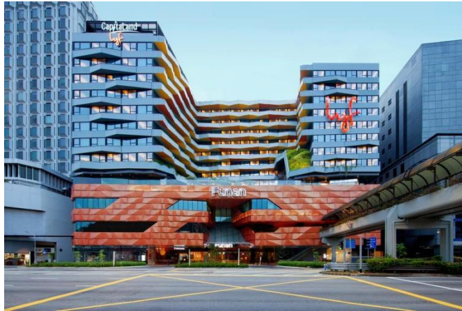
PLATE 21: 3V view of Funan Mixed use complex Source - (Google search)
