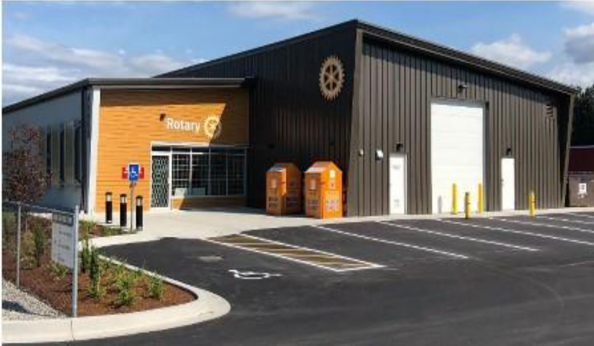
Figure: 3.13: Rotary Club House International- Chilliwack Canada, showing lighted environment (Source: www.rotary.org )
