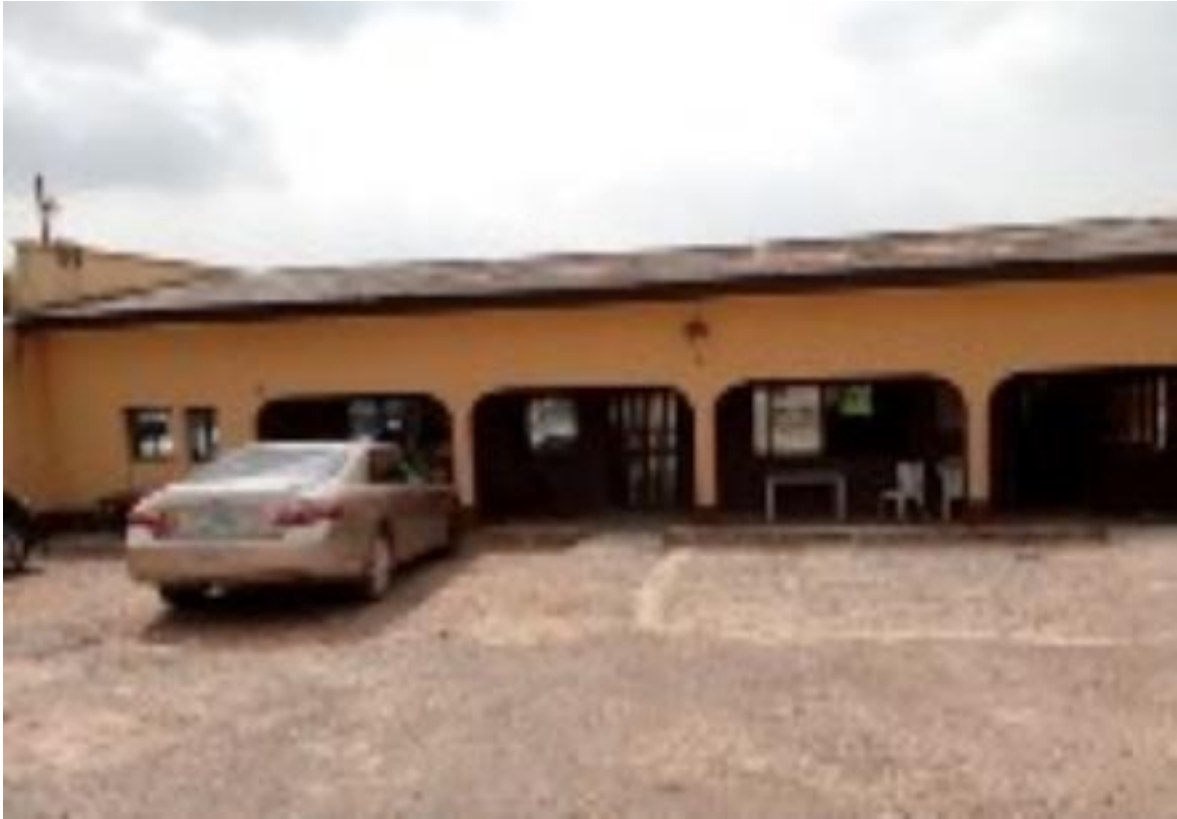
Fig 3.24. NUJ Conference Hall Side view (Source; Author's field work)
