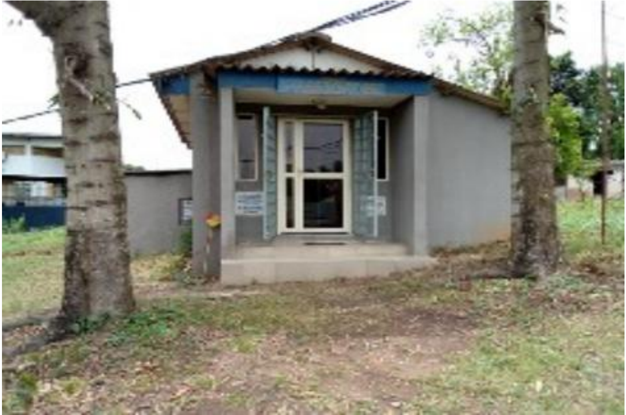
Figure 3.22. Administrative block Approach Elevation, Rotary Club House –Ibadan (Source: Author’s field work)
