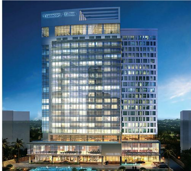
Figure 3.5.1: view of Transcorp Hilton-Lagos Nigeria Source: The Author
