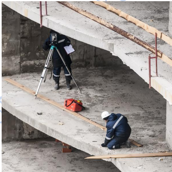
Figure 2.7: Site construction workers Source: The Author
